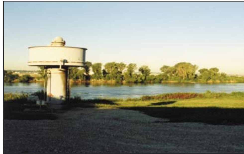
Wells located along the Missouri River supplement water from the river with water from the aquifer. The well water helps to maintain consistent water temperature throughout the year.
