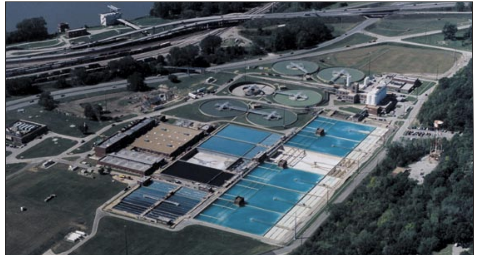
The Kansas City, Missouri Water Services Treatment Plant was constructed in 1925 as a modern innovation in water treatment and was the City's largest capital expenditure when built. Today, the plant has a capacity to treat 240 million gallons per day.
