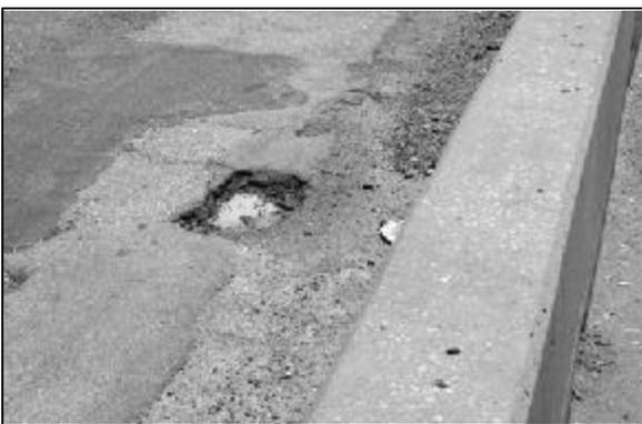
This section of N Brighton (on the bridge over I-35) continually has potholes
