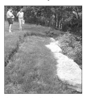
The resident pictured above lives upstream from the North Lakes drainage lagoon. The resident built a rock retaining wall to stop erosion of the channel that runs along the side of his home. Despite his efforts the portion of his yard that abutts the channel has dropped several feet.
