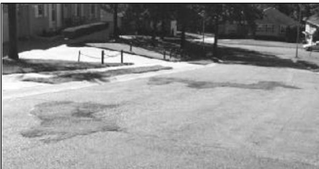
Residents would like to see the insufficient water mains replaced (they are the cause of these potholes), rather than seeing the potholes filled over and over
