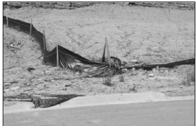
When erosion controls are ineffective, soil builds up on streets and runs into storm sewers
