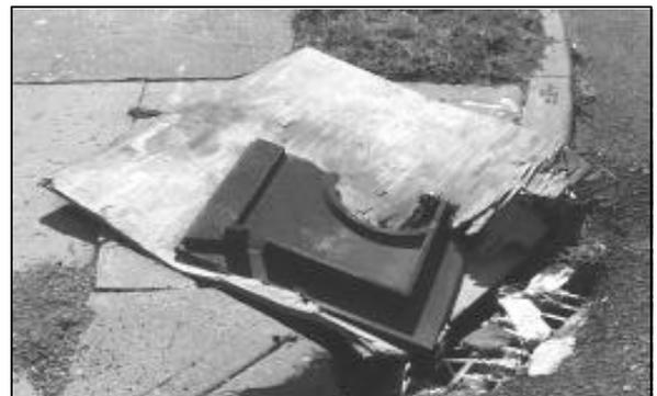
A broken catch basin on the northeast corner of 63<sup>rd</sup> and Harrison.
