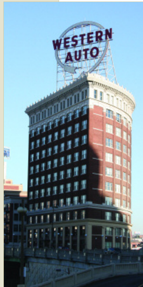
The Western Auto building loft conversion was one of the first large-scale residential projects Downtown.
